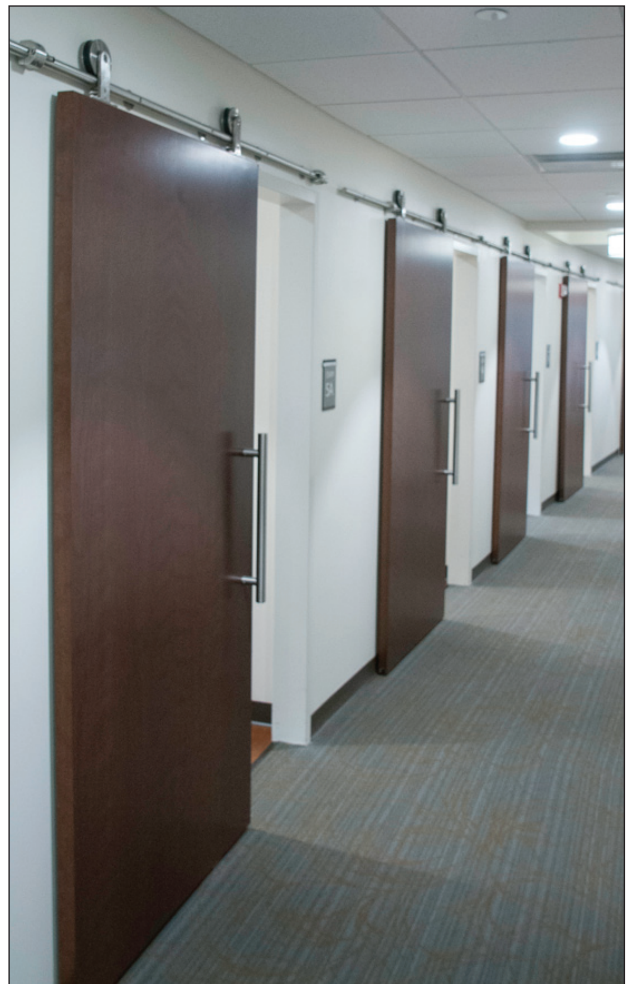
Figure 1. Designing a space with doors that sit on sliding rails saved enough room to add 14 new examination and treatment rooms.
